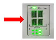
**STEP 3:** Wait (about 10 seconds) until the USB Detected light on the wall shines, then turn TV Preview on.
